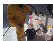
STEP 3. Saturate the pool shell thoroughly with water. Always keep it saturated during the acid wash process. This helps prevent depth of penetration, overexposure of the aggregate and degradation.
