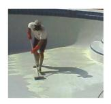
STEP 10. Carefully pressure wash the surface of the pool to remove film and any remaining pasty areas. Exercise extreme caution to not damage the finish. If there are any remaining paste areas Poof may be used moderately.
