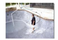
STEP 4. After saturating the pool surface leave the water in the bowl to help neutralize the acid.
